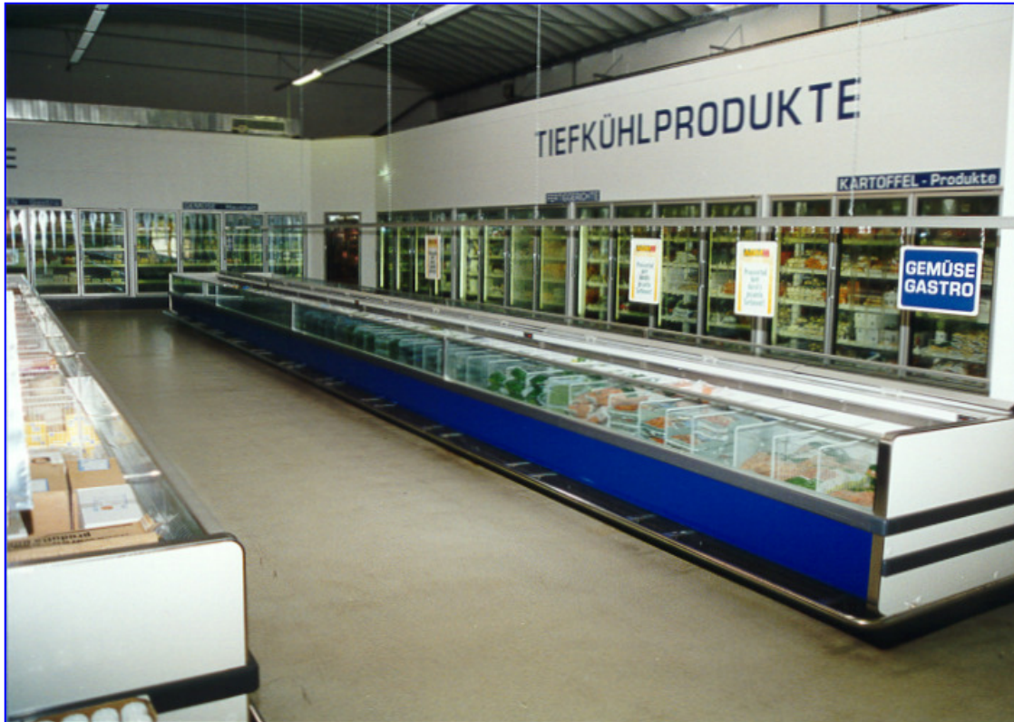
Sales room of a hypermarket—glass doors for the deep-freeze cabinets with combined storage facilities and loading of the shelves from the back.
